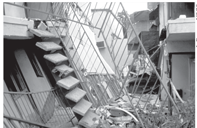
Figure 36 - Stairs to an apartment building collapsed during the 1994 Northridge earthquake.
