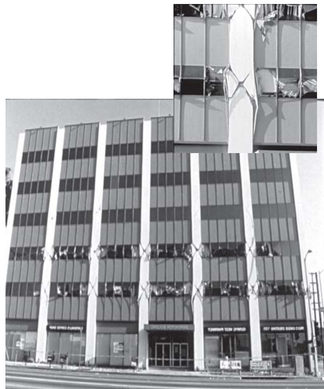
Figure 23 - This medical office building's exterior cladding affected the way its frame responded to shaking, and the columns failed during the 1994 Northridge earthquake. The building was demolished and all medical records inside were destroyed.
